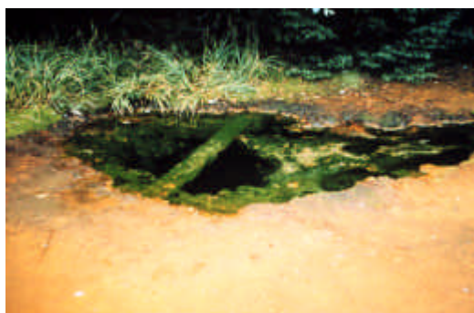
Figure 4. Mine portal, Maryland
